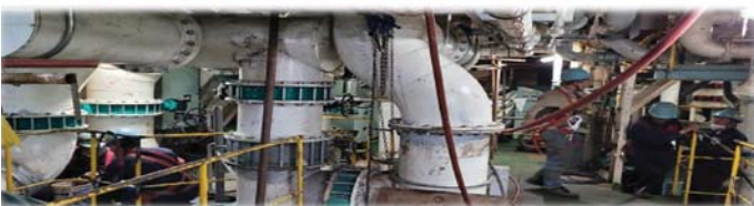
A new ballast water treatment system was installed and commissioned by Techcross and was a major work undertaken during the repair period.
